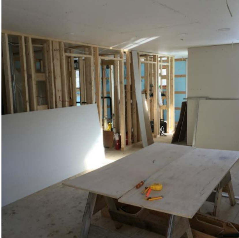
Photo: NLC Staff Housing project progress
